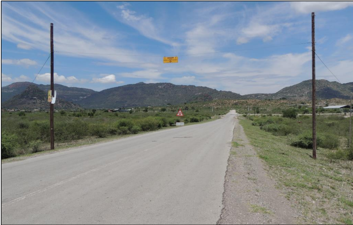
Figure 14. Photograph of the Marula Platinum Mine access road which would be used by mining vehicles as well as rural residents.
