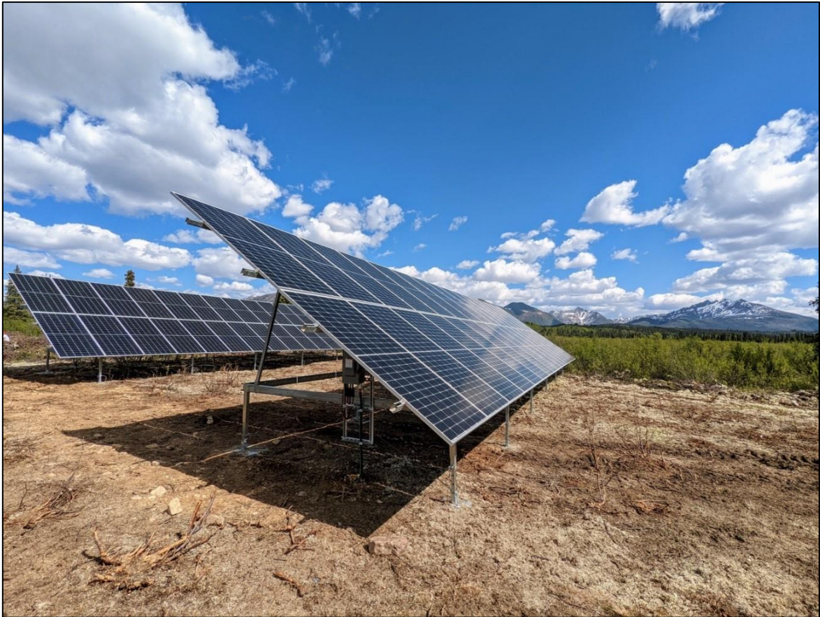
Figure 3: Photographic example of what the proposed PV could look like as fixed and single portrait model on a tracker.
