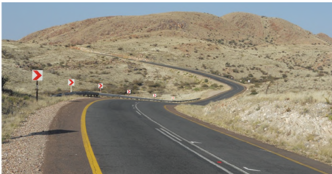
Figure 1: N10, kilometre chainage 87.2
