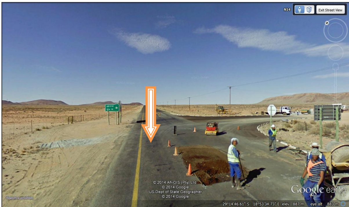
Figure 2-3: Proposed access point to Namies Suid/ Poortjies site adjacent to N14 – street view
