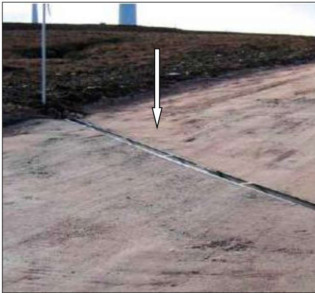
Figure 2-3: Cross drains under the Internal Roads
