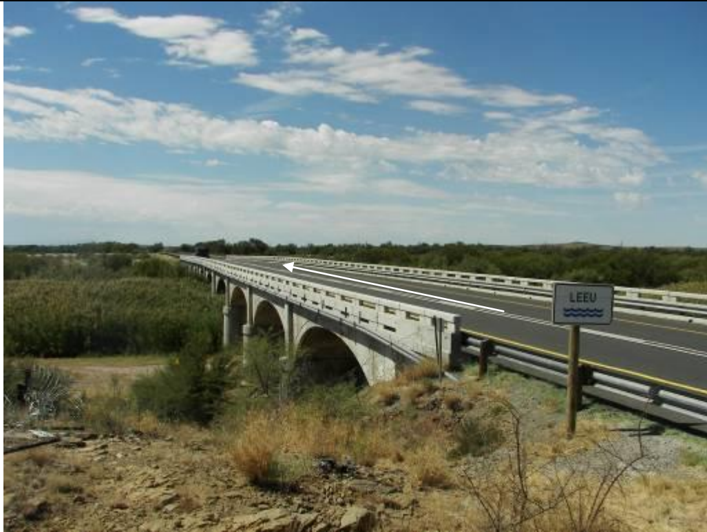
Bridge 4918 over the Leeu River on the N1 (Typical)
