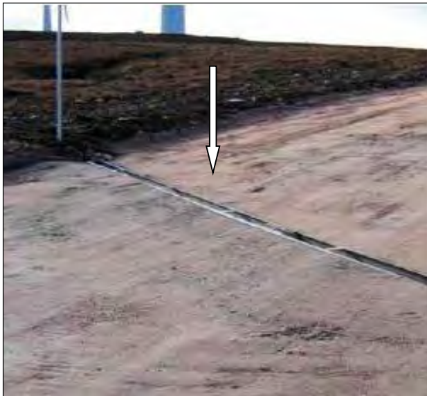
Figure 2-3: Cross drains under the Internal Roads
