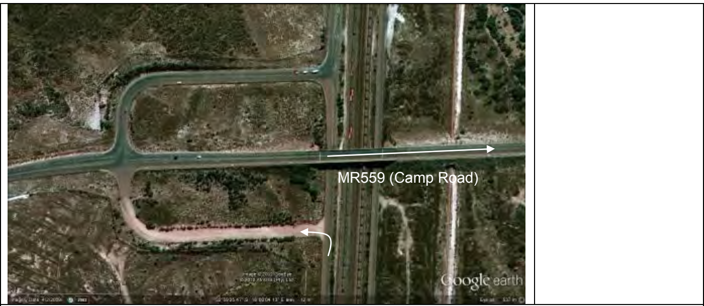
Overview gravel ramp onto MR559 (Camp Road)
