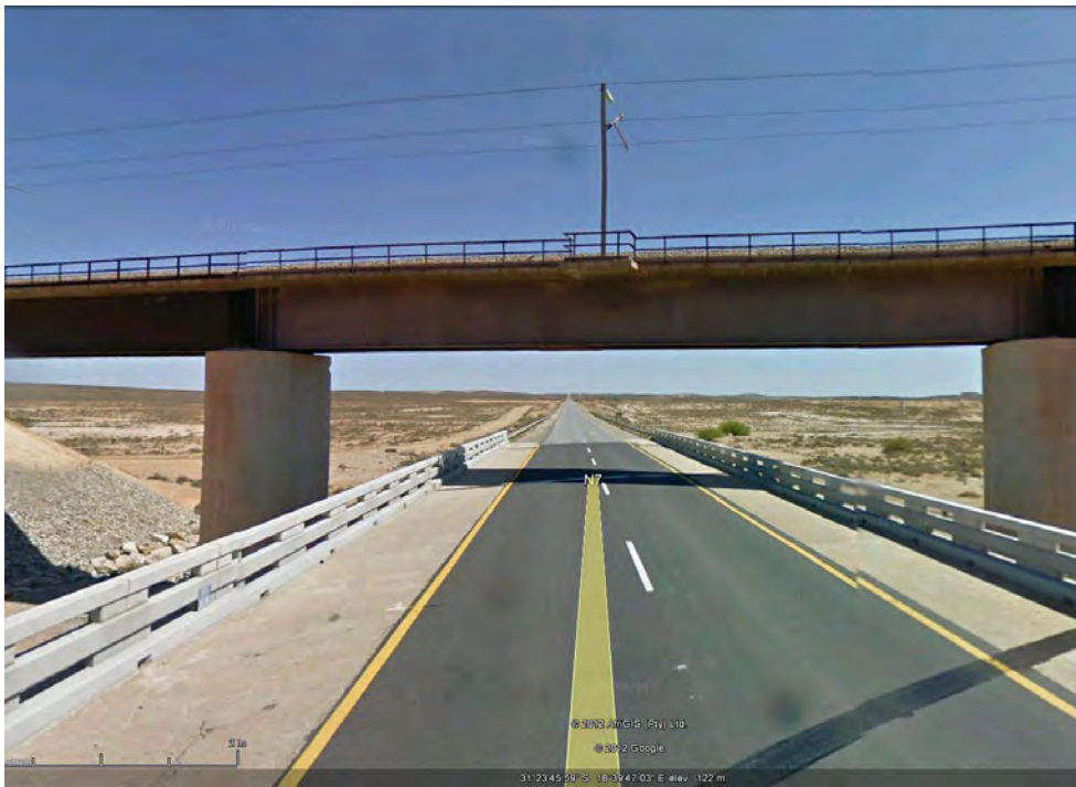
Overhead Railway Bridge on N7, Vanrhynsdorp
