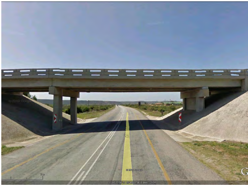
Overhead bridge on the N2 at Cannonville, just past the Sondags River
