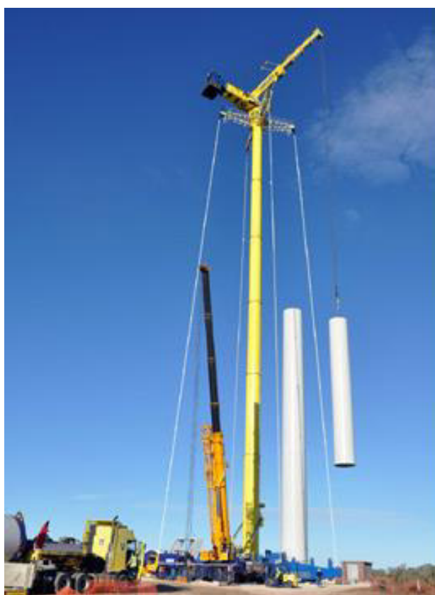
Figure 2.6: Example - Cranes at work
