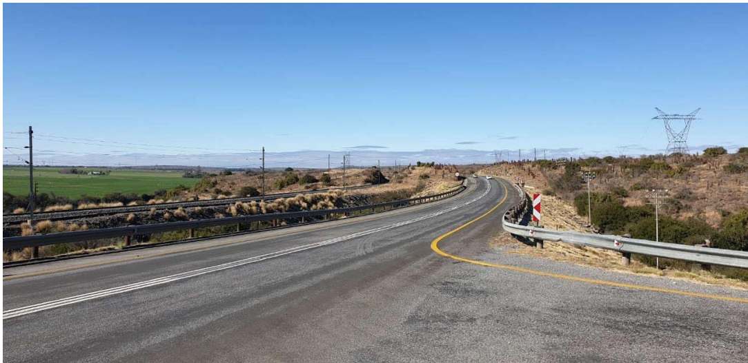
Figure 3-6: N10 Southbound at Access Point 2
