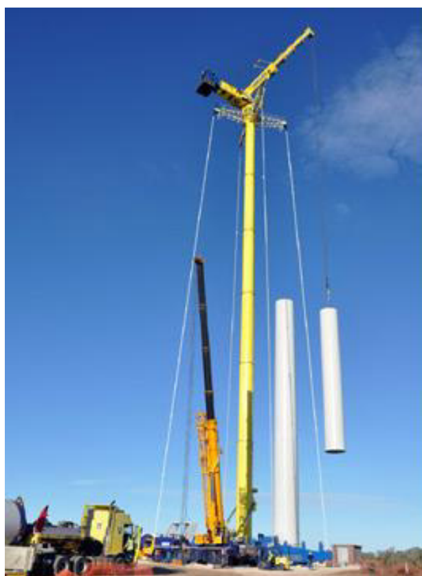
Figure 2-6: Example - Cranes at work
