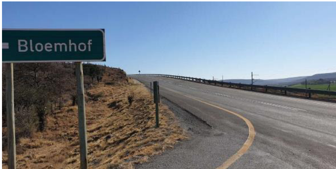
Figure 3-8: Limited sight lines in northbound direction on N10
