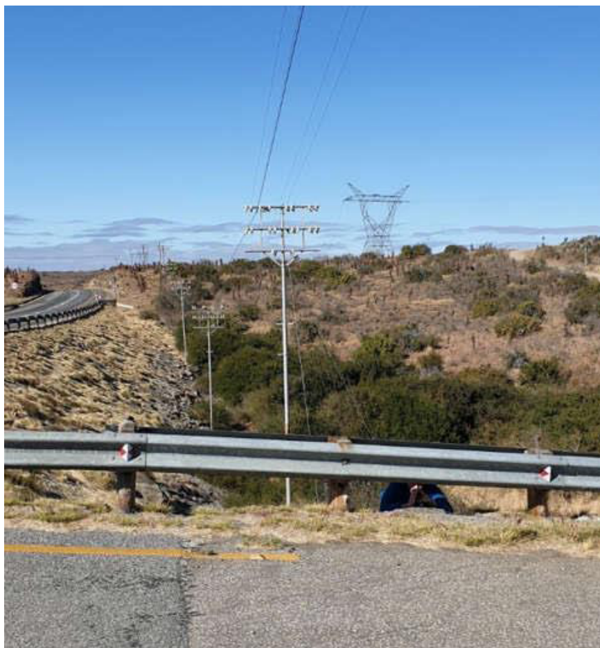
Figure 3-7: Overhead lines at Access Point 2
