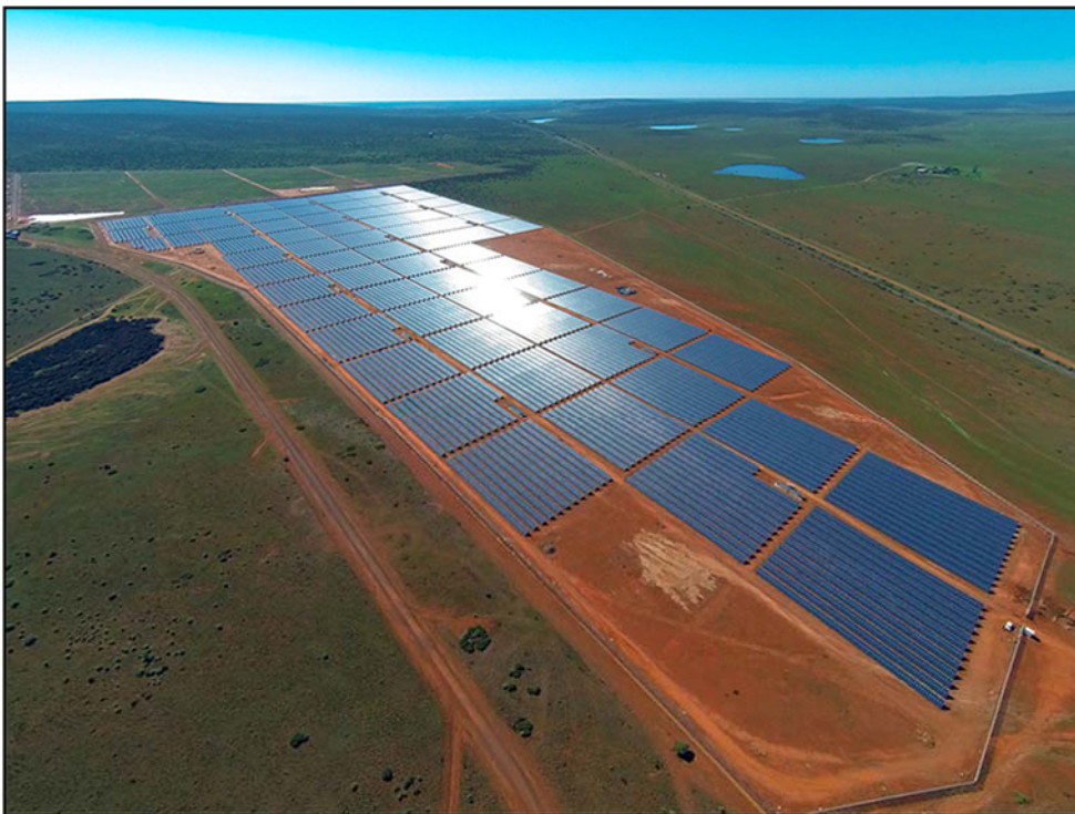
Figure 1-1: The Lesedi Solar Park near Postmasburg in the Northern Cape. This solar park is an example of a Photovoltaic (PV) Solar Power Plant 1
