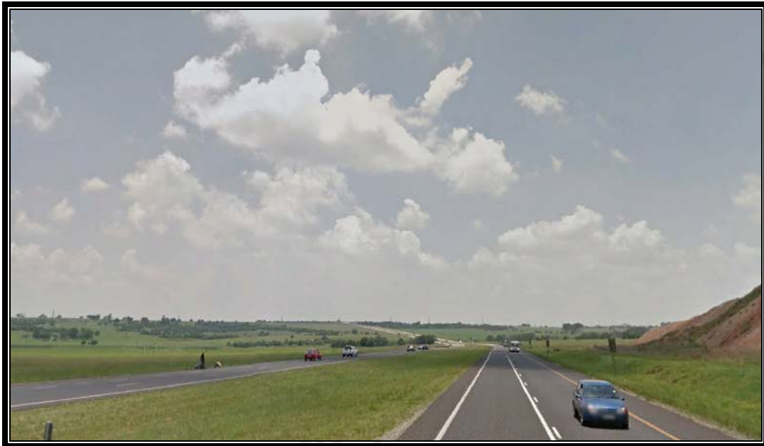
Figure 4: Road R545 across the N12 freeway
