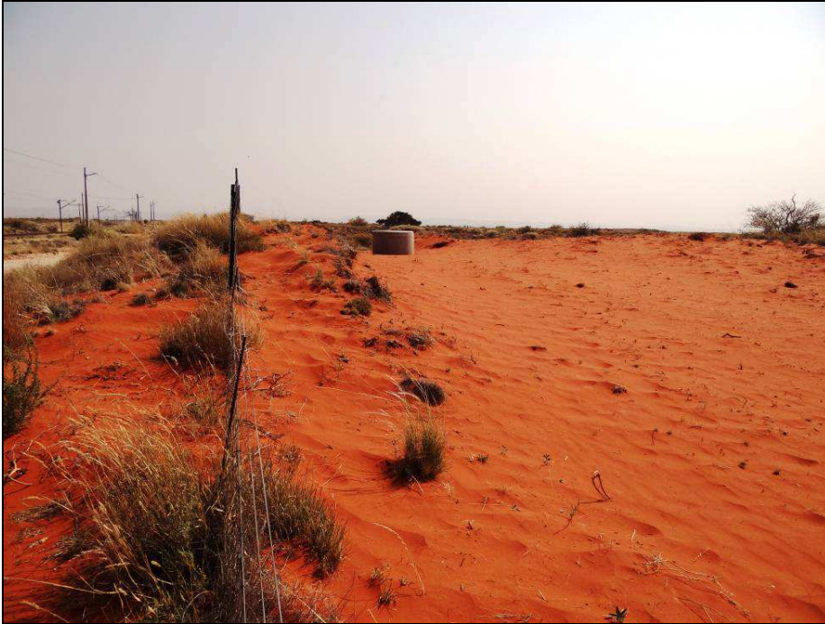
Fig.14 Point P2 on the existing water pipeline to Garona Sub-station.
