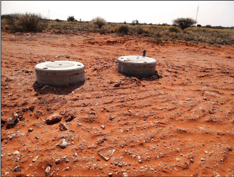
Fig.12 Point P1 along the existing water pipeline to Garona at Bokpoort.
