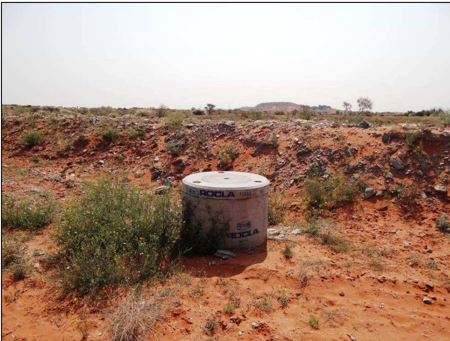
Fig.13 Point P1 along the existing water pipeline to Garona at Bokpoort.
