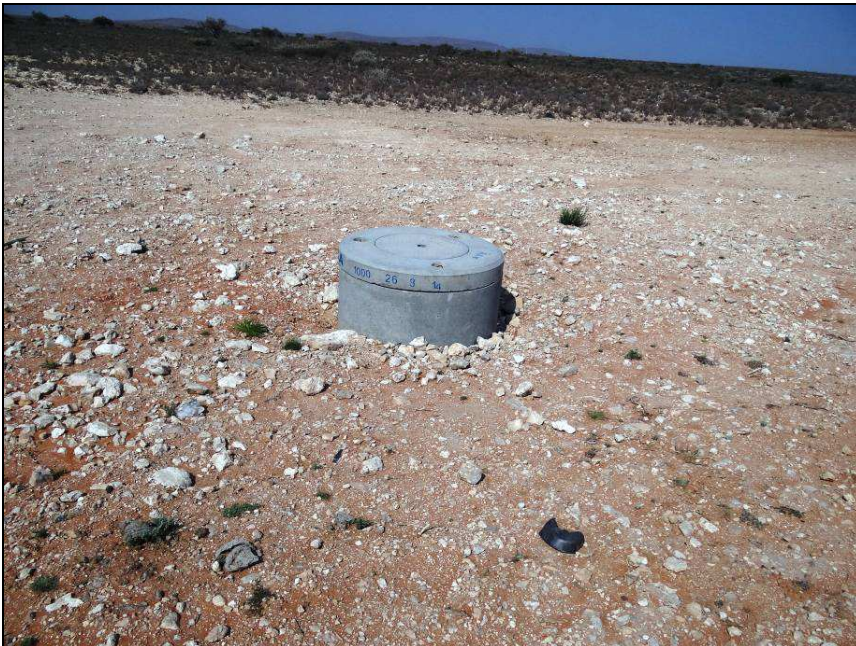
Fig.17 Point P4 on the existing water pipeline to Garona.
