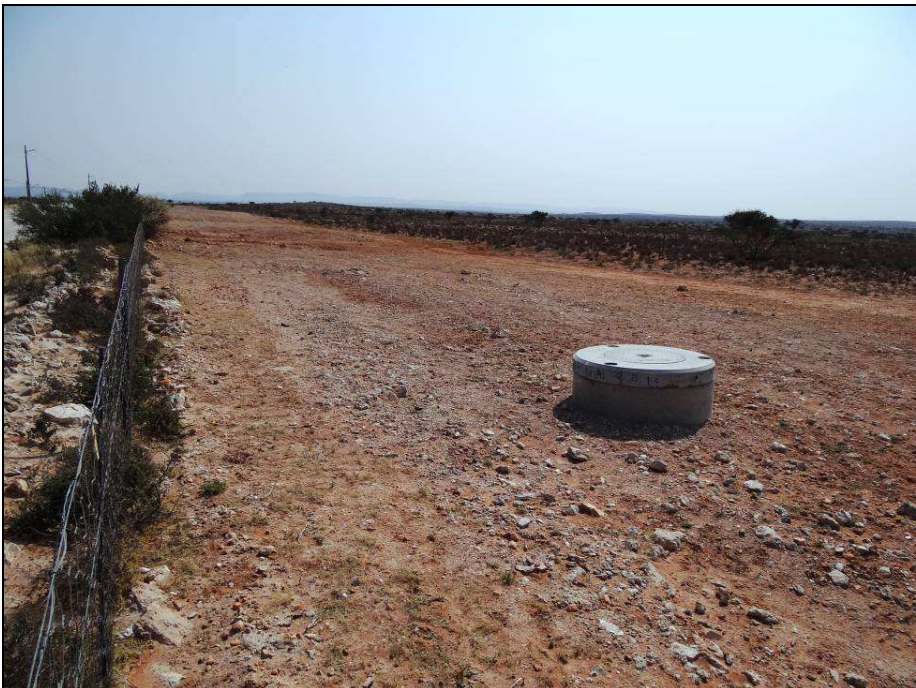
Fig.15 Point P3 on the existing water pipeline to Garona.
