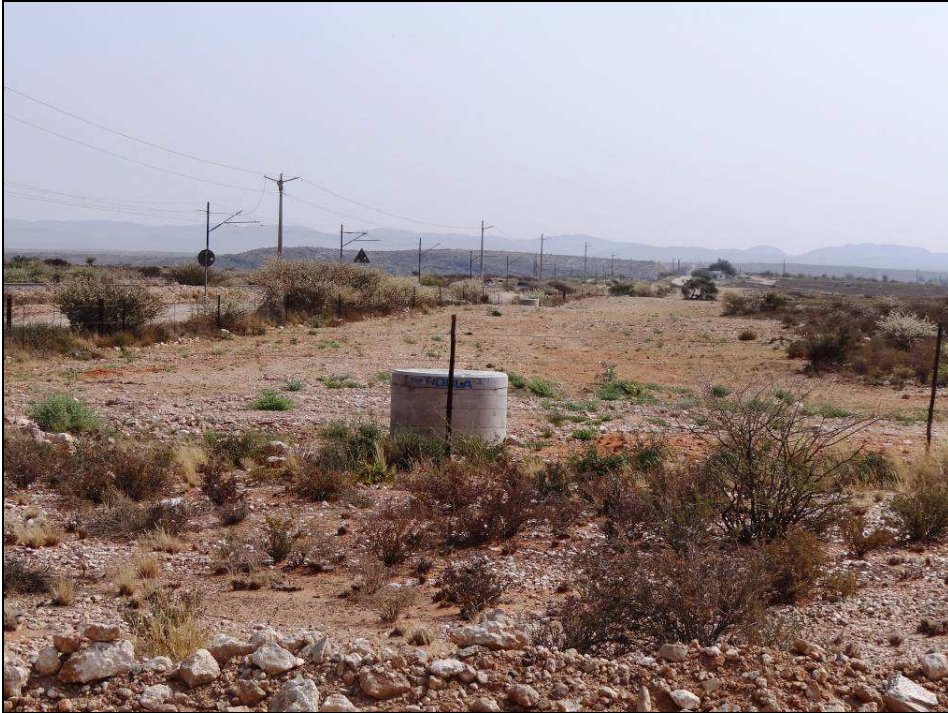
Fig.18 Point P4 on the existing water pipeline at the railway crossing to Garona.
