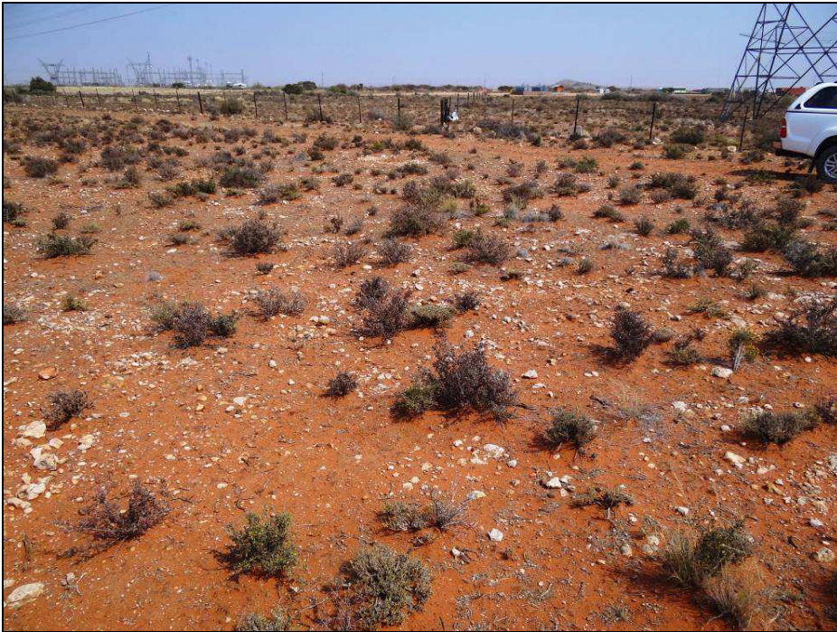
Fig.2 Point E at Bokpoort II, Groblershoop. Garona Sub-Station on left of picture.
