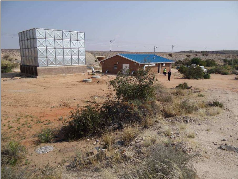
Fig.20 Existing water pump station near Point P5 on the pipeline to Garona Sub-Station.
