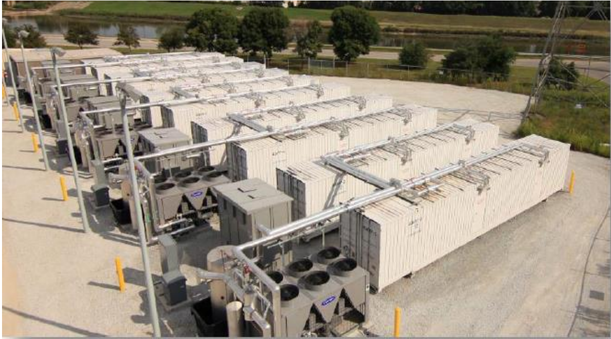
Figure 3-4: Example of a Solid-State battery facility layout
