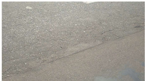
N1/D1021 intersection (looking north along N1)
