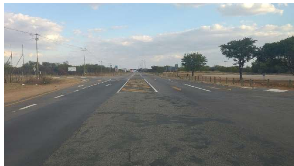
N1/D777 Intersection (view south along N1, towards the Boabab Toll Plaza)
