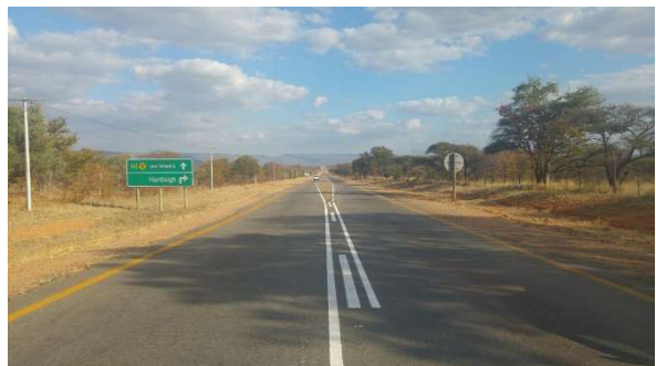
N1/D1021 intersection (looking south along N1)
