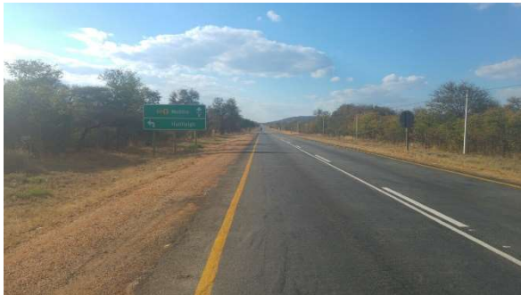
N1/D1021 intersection (looking north along N1)
