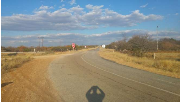
D777 looking east towards rail level crossing
