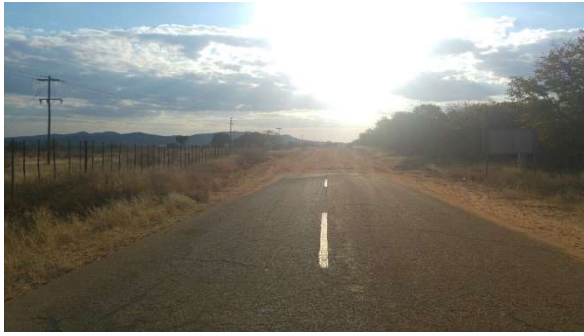
D777 looking west from D744 intersection
