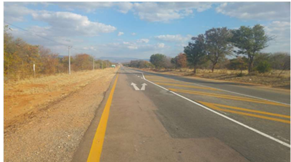
N1/D1021 intersection (looking south along N1)
