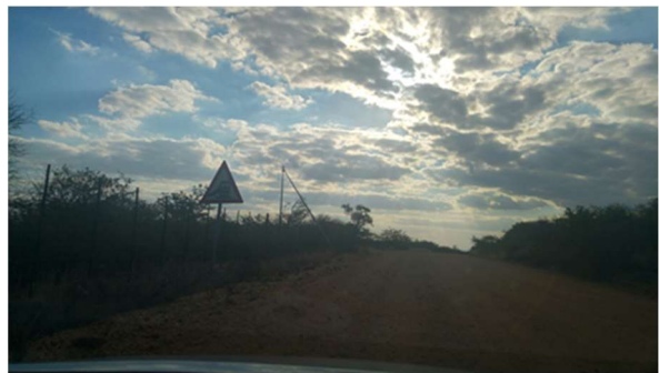
D1021 - railway line level crossing warning signage
