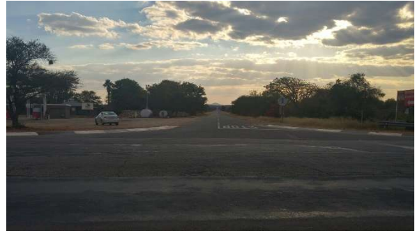
N1/D777 Intersection (view from N1 along D777)
