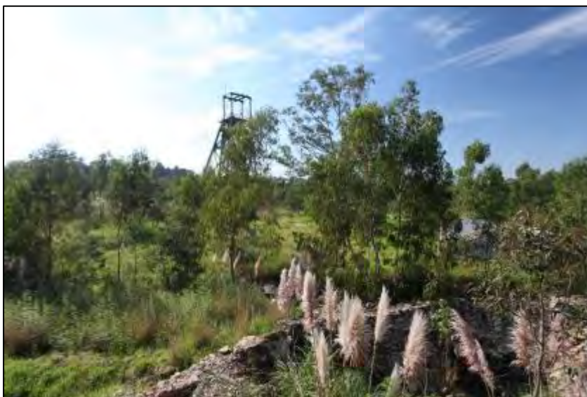
Figure 9: General view of the Bird Reef Central Infrastructure Complex (IC) indicating a shaft, remnants of historic mining infrastructure and dense vegetation of the area.
