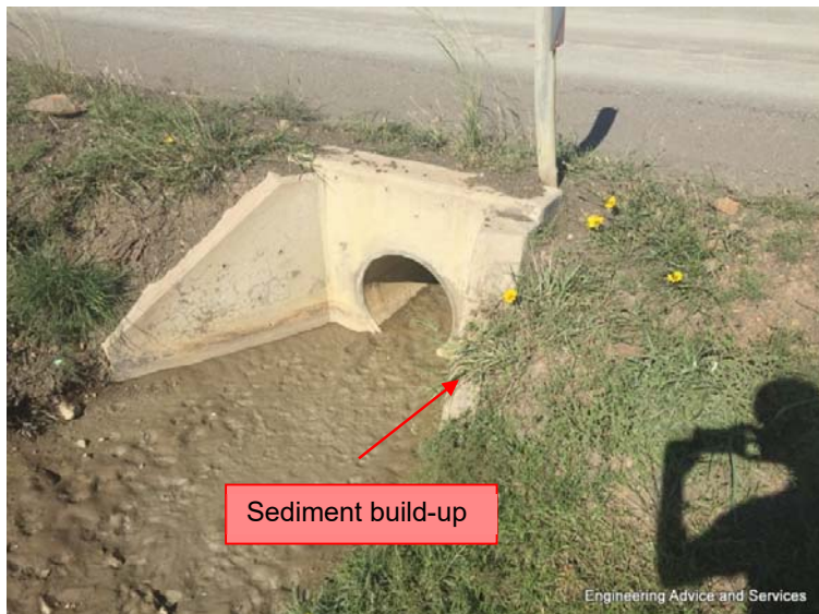
Figure 4 – Typical Stormwater crossing along MR00481
