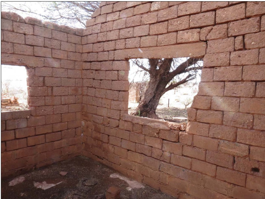
Figure 34- Sample of walling showing the mud bricks used to construct the homestead.
