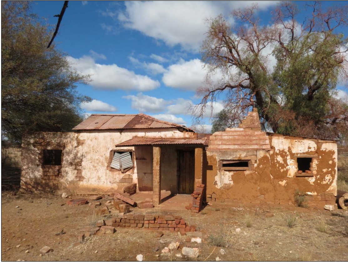
Figure 35 - Northern façade with small veranda and back door.
