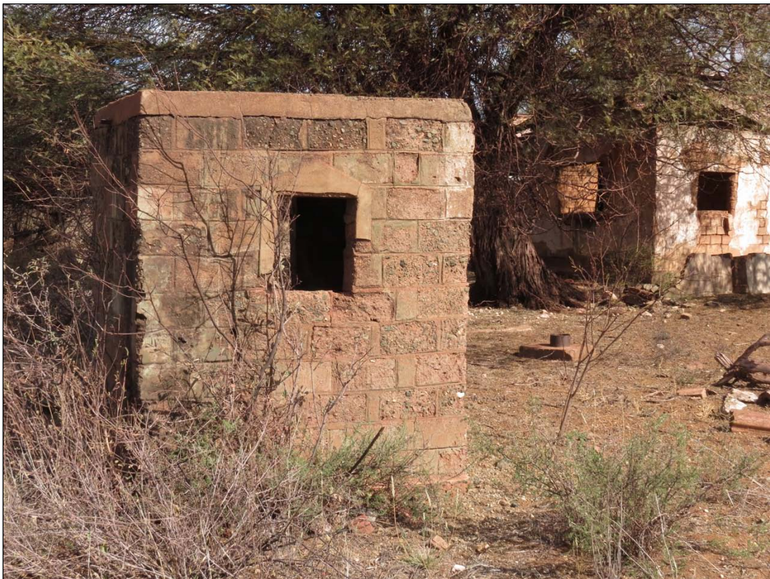
Figure 36 - The outside toilet with a section of the house visible in the back.
