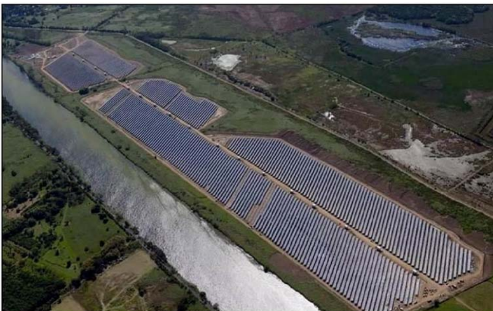
Figure 2: Example of a single axis tracking photovoltaic (PV) solar power plant
