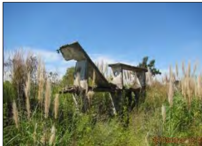
Figure 60: View of remains of structures
