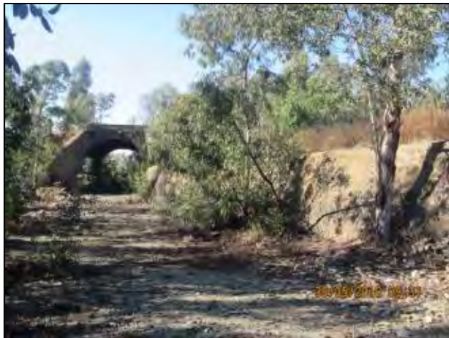
Figure 61: View showing the long structure (right hand side) and associated tunnel
