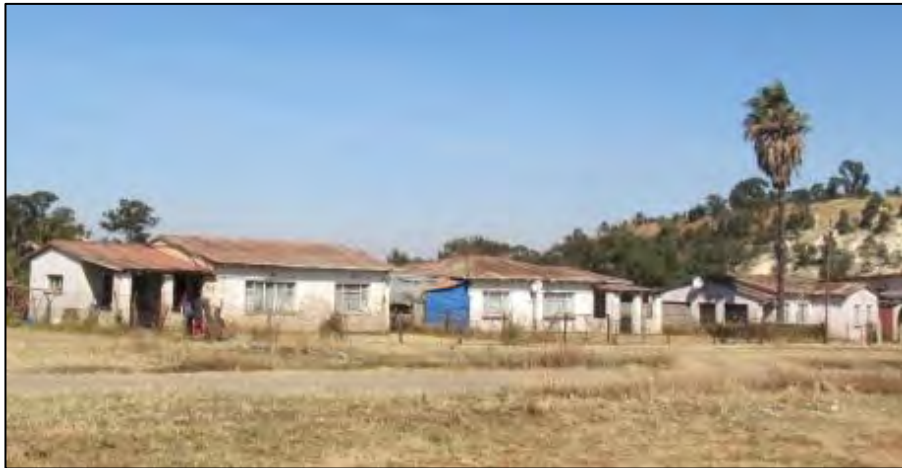
Figure 108: Site WW023, view of historical houses
