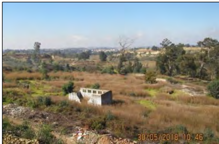
Figure 67: WW009 and WW009-1, general view showing the structure remains and foundations
