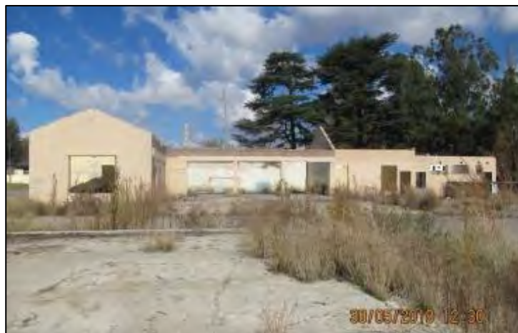
Figure 76: WW012, view of the structure remains with foundations
