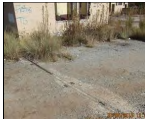
Figure 77: Closer view showing a section of rail
