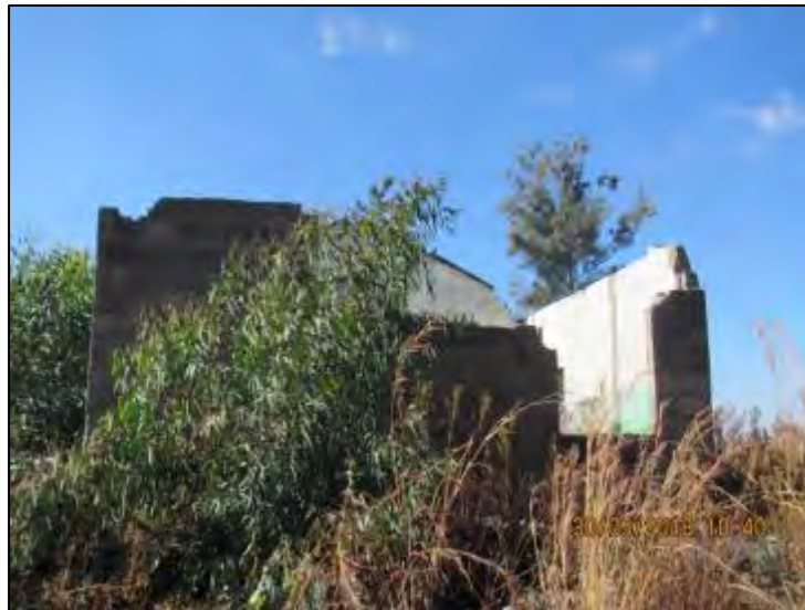
Figure 66: WW-008, view of small structure at top of waste rock dump
