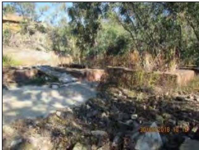
Figure 64: View of the demolished structure
