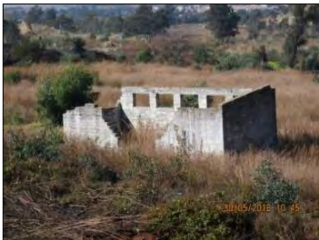
Figure 68: Closer view of structure remains
