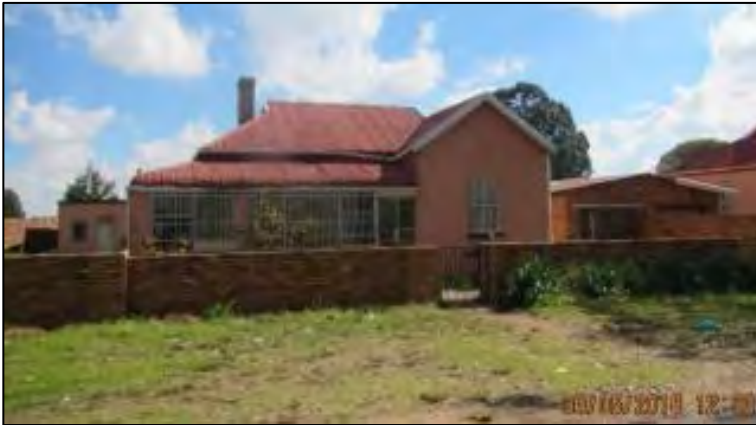
Figure 79: View of a house with a single gable
