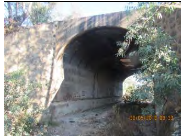
Figure 62: View of the rear of the tunnel
