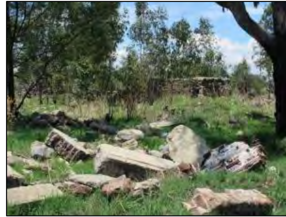
Figure 87: View of ruined structure and building rubble
