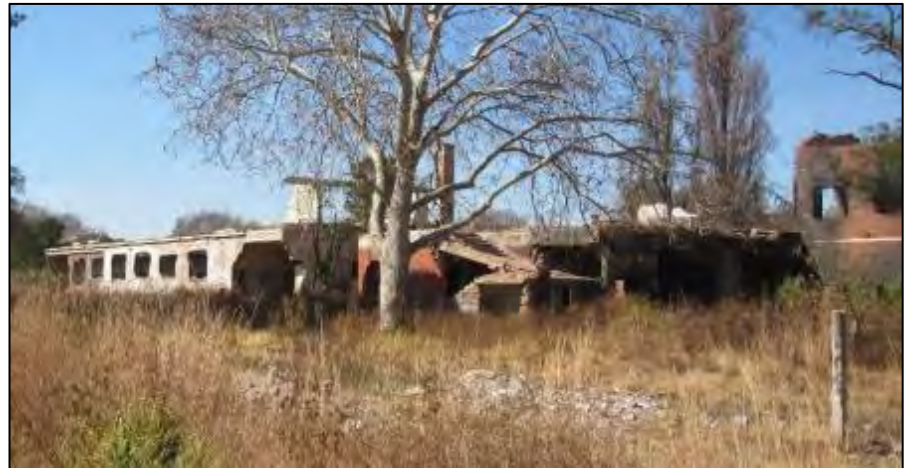
Figure 109: View of dilapidated large double-storey building
