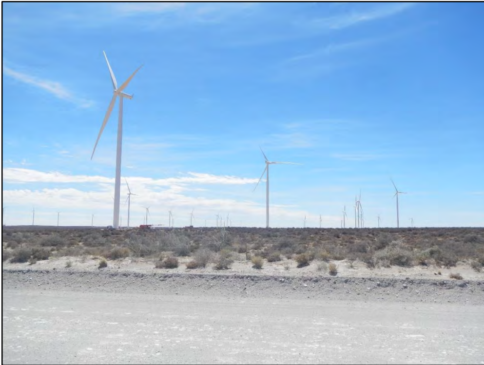
Figure 19: Wind turbines at the Loerisfontein Wind Farm.
