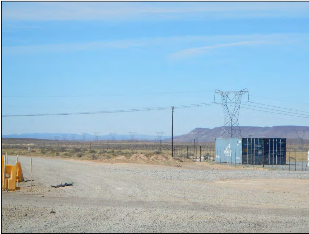
Figure 18: High voltage power lines feeding into Helios Substation.
