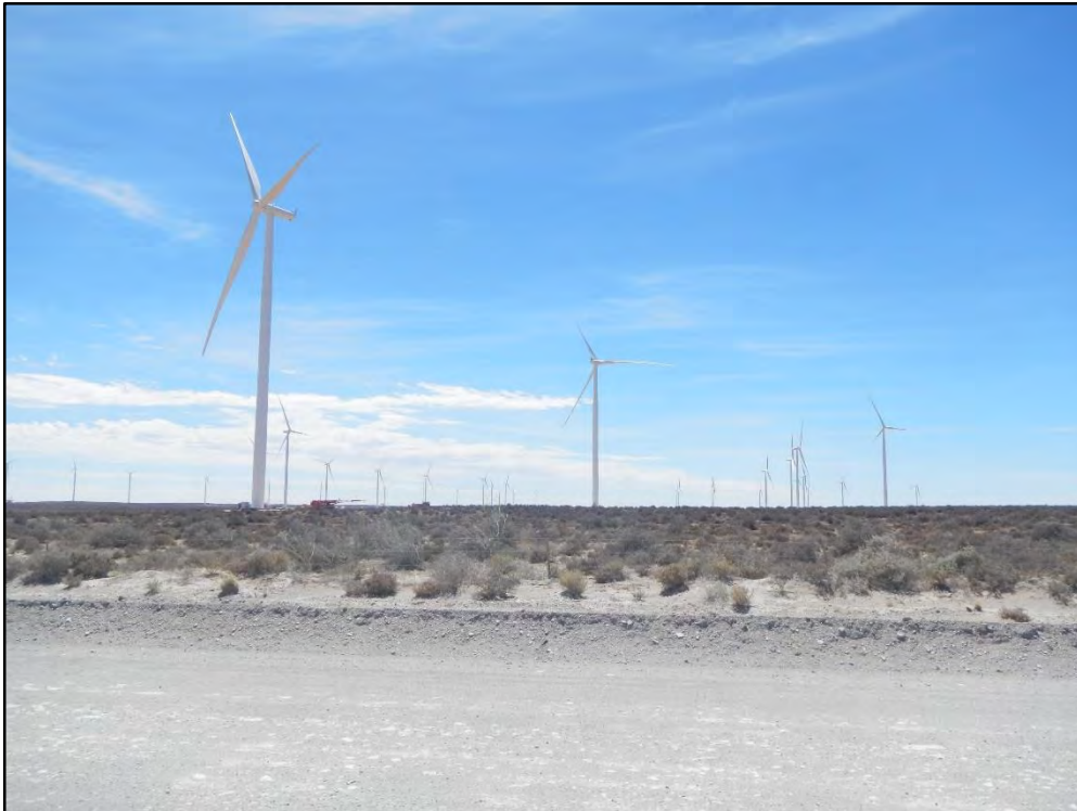
Figure 19: Wind turbines at Loerisfontein Wind Farm
