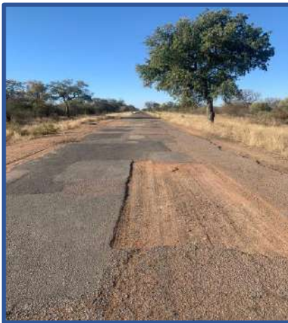
Photo 1: D1675 looking west
