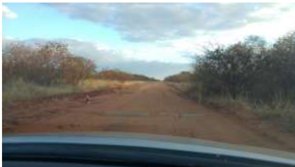
D744 - Exposed culvert
