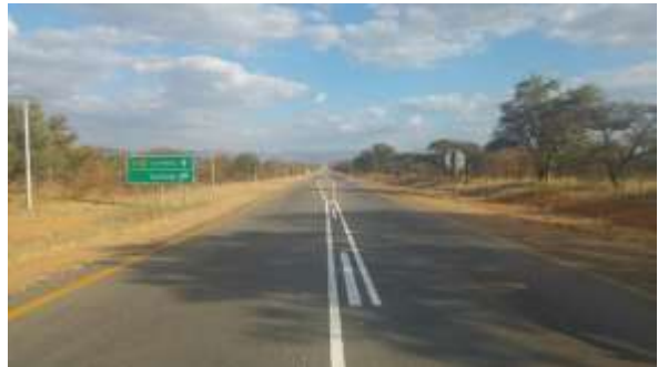
N1/D1021 intersection (looking south along N1)
