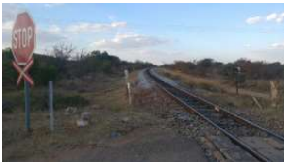
Level crossing on D777 in Mopane viewing north
