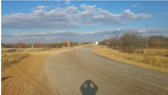
D777 looking east towards rail level crossing
