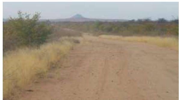
Inside horizontal curve viewing to north
