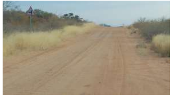
D744 Vertical alignment restricting sight distance viewed towards D102
