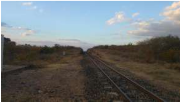
D1021 - Sight line to north at rail level crossing limited by narrow cutting and rail line geometry
