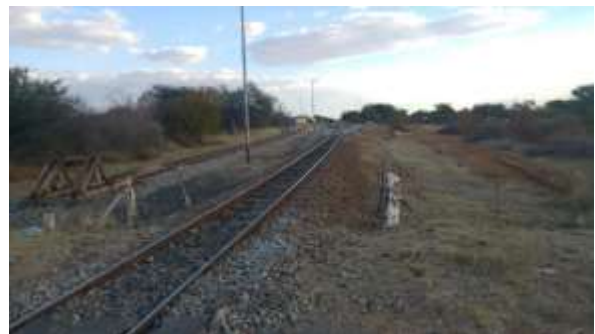
Level crossing on D777 in Mopane viewing south
