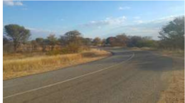
D777 looking west towards Mopane from rail level crossing
