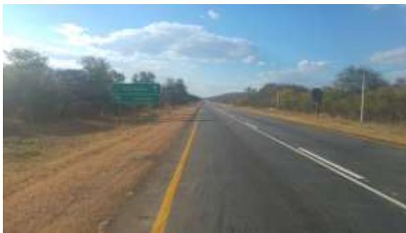
N1/D1021 intersection (looking north along N1)
