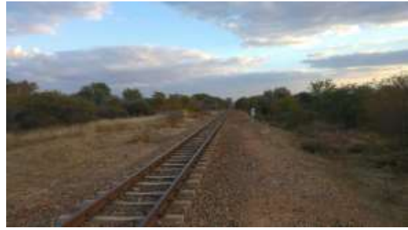
D1021 - Sight line at rail level crossing ok to south
