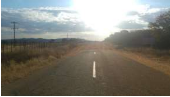
D777 looking west from D744 intersection
