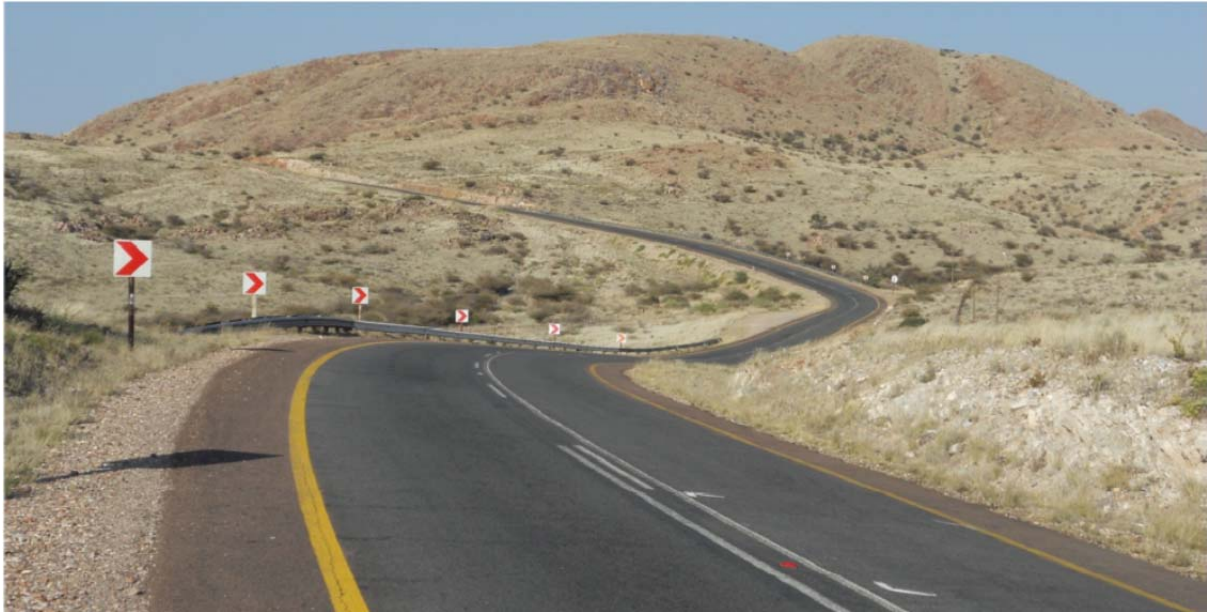
Figure 2: N10, kilometre chainage 87.2
