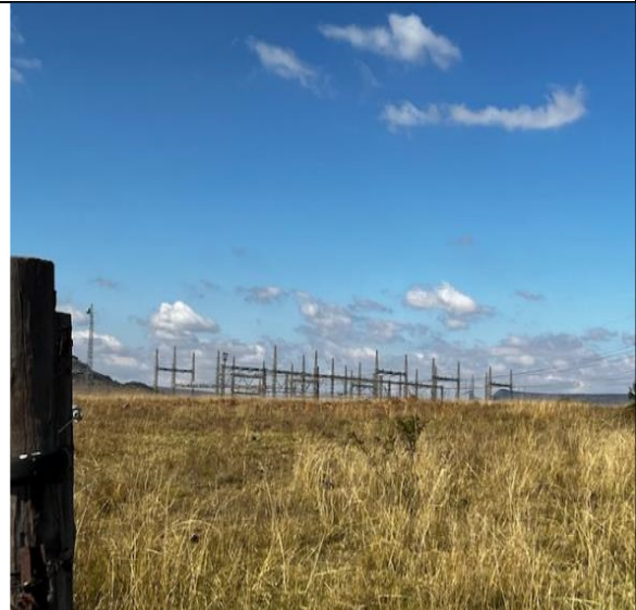
View of the existing Bloedrivier Substation
