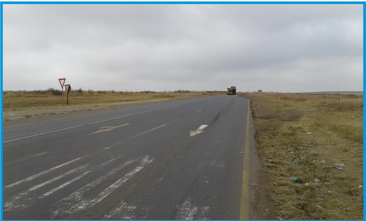
Photo 2: R545/R547 Intersection – East Approach
