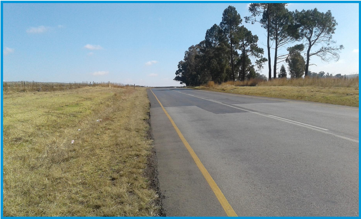
Photo 13: Sight Distance West of Proposed Access
