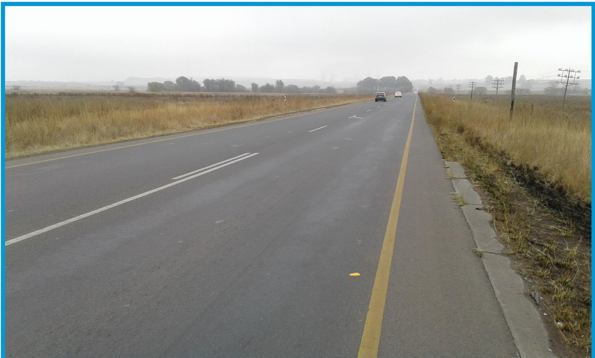
Photo 6: Road Surface along R545, West of Kriel – Generally Good
