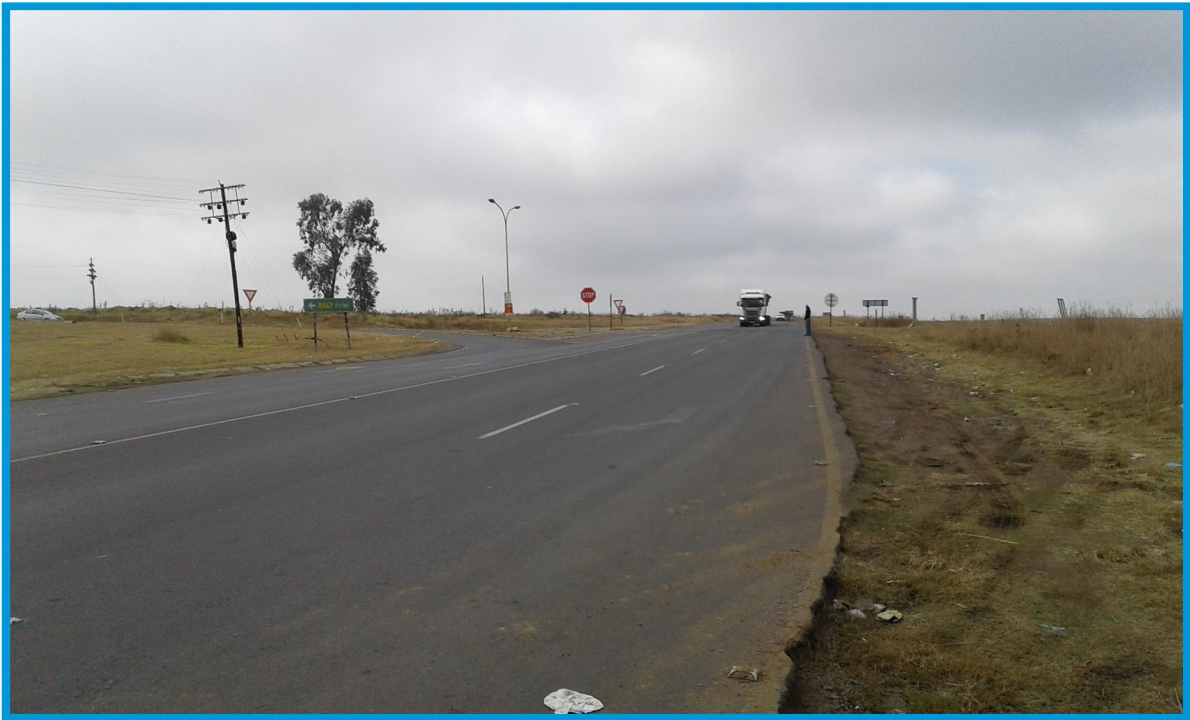
Photo 3: R545/R547 Intersection – West Approach
