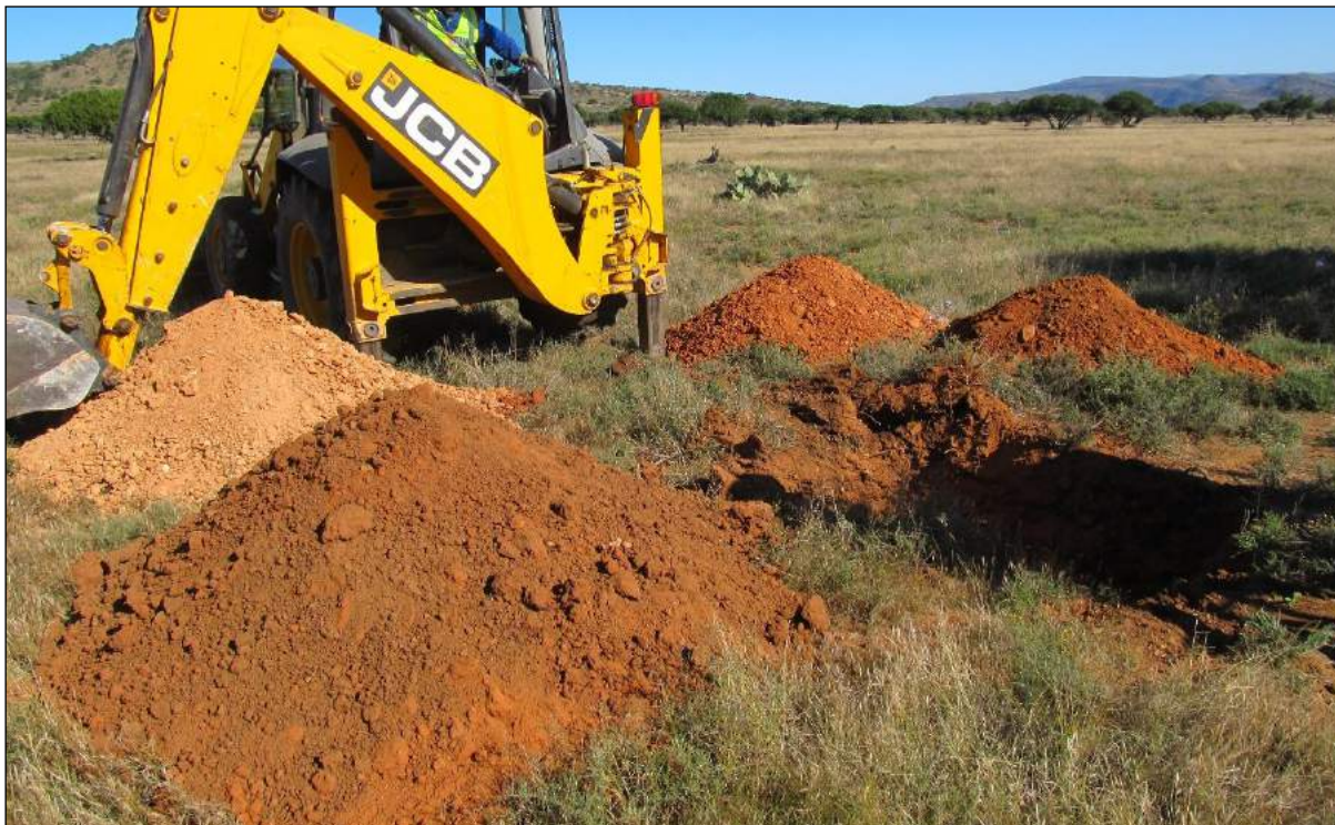
Plate 2: Trial pit excavation at W417 position (photo credit: Outeniqua Geotechnical Laboratory)
