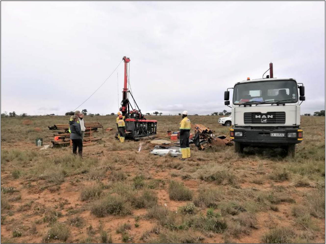
Plate 1: Rotary core drilling at borehole position E64
