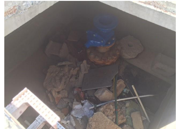
A man-hole occurring at the upper reaches of the wetland.
