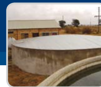
Seamless Concrete Reservoirs Gunite Dam
