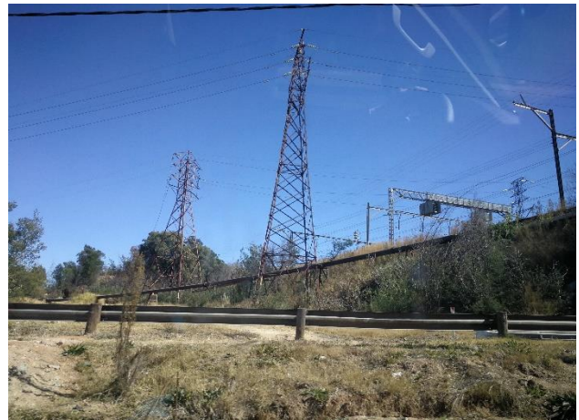
Figure 1-6: Infrastructure found in the project area including pipelines and powerlines.
