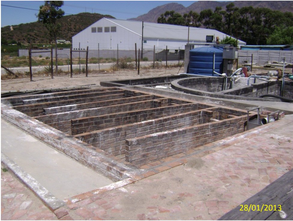
Photo 1: Existing Montagu Cellar Waste Water Treatment Works to be upgraded and expanded.
