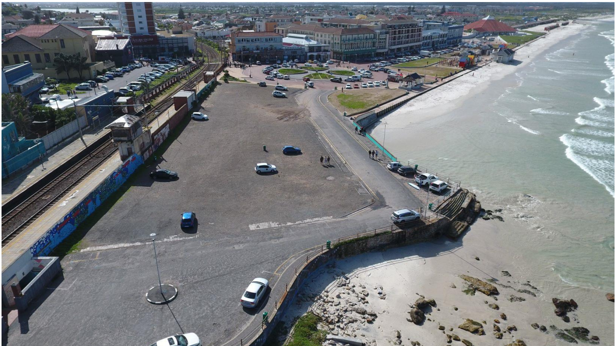
FIGURE 12: Gravel parking facility and the "Point"
