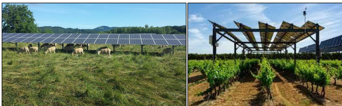
Figure 25: Depicts an agrivoltaics or agrophotovoltaics systems used to co-develop the same area of land for both solar photovoltaic power as well as for agriculture in order to possibly reduce the loss of land capability and land potential.
