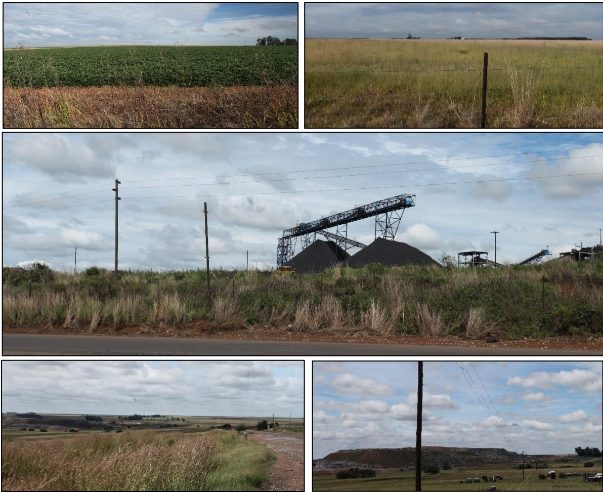
Figure 4: General view of the study area and surrounding area indicating the agricultural crop fields (top left), active mining activities and grassland (top right), existing overhead powerlines and active mining activities along the proposed powerline route (middle), and grassland and a mine dump in along the proposed powerline route (bottom left and right).
