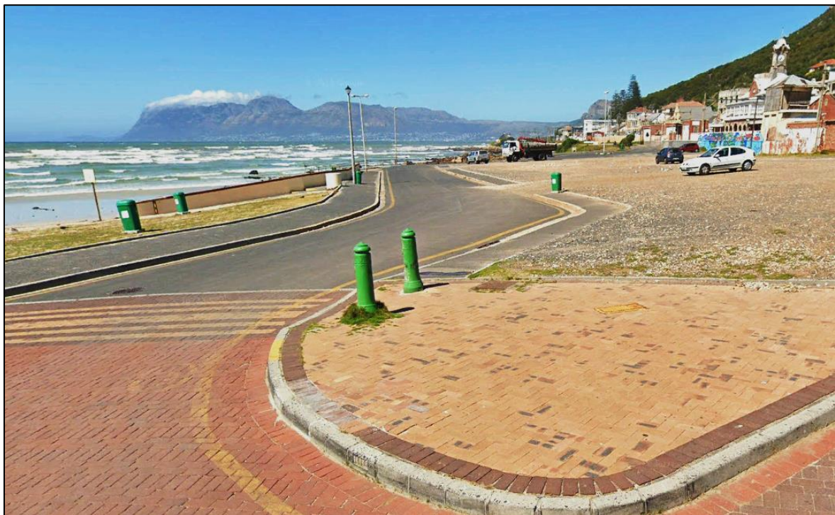
Figure 2-2: Existing Access from Traffic Circle to Informal Parking Area
