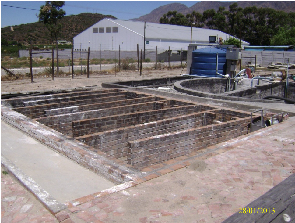
Photo 1: Existing Montagu Cellar Waste Water Treatment Works to be upgraded and expanded.
