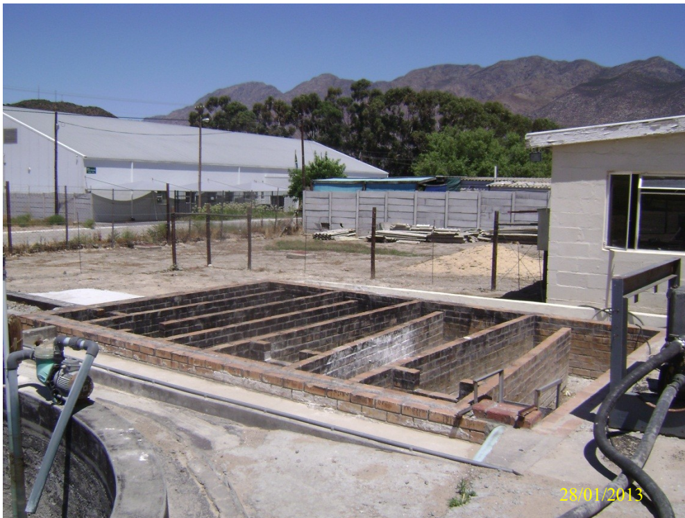
Photo 2: Existing Montagu Cellar Waste Water Treatment Works to be upgraded and expanded.
