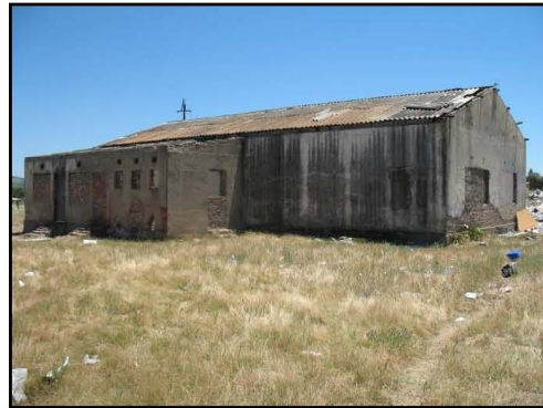
Figure 11. Back of the building
