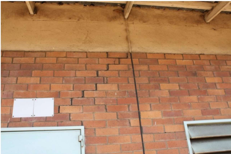
Figure 8: Example of blast induced damage.
