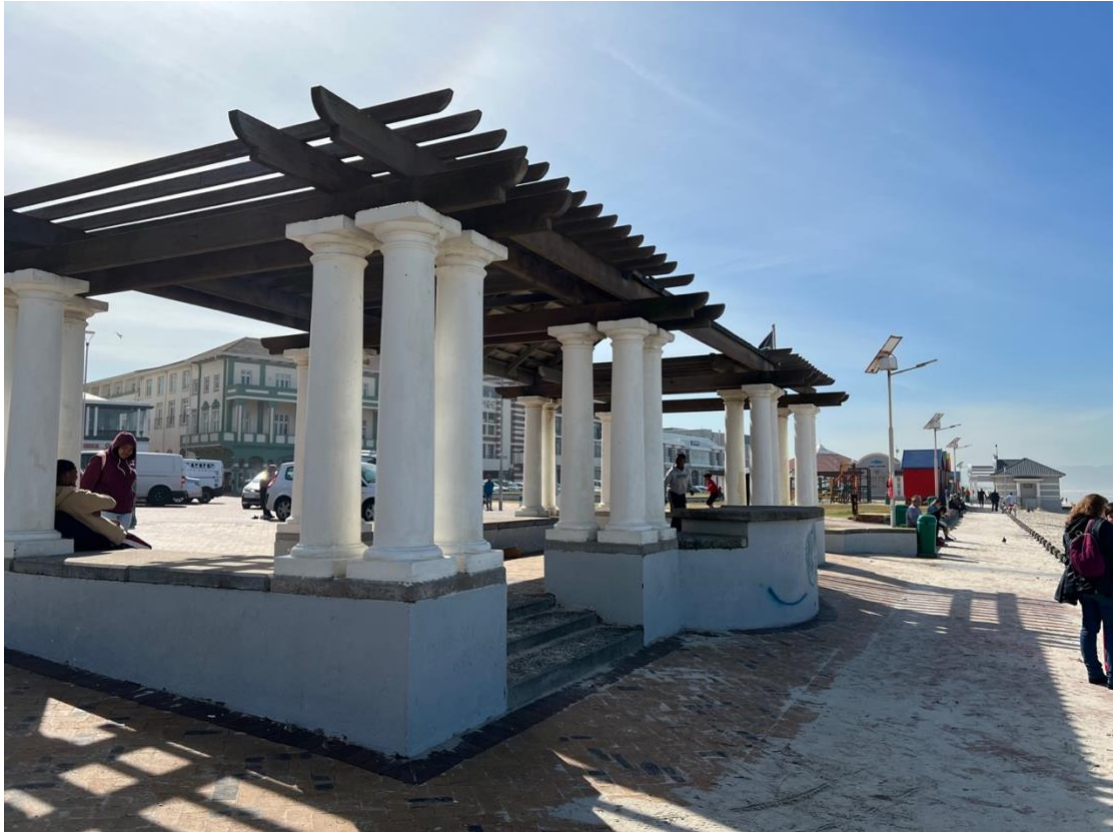
A North-East facing view of the site showing the extensive development
