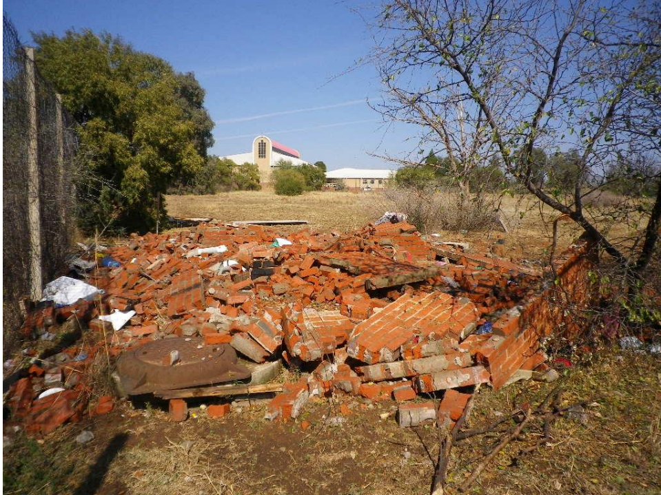
Photo 7: Remains of a dilapidated building still present on site.
