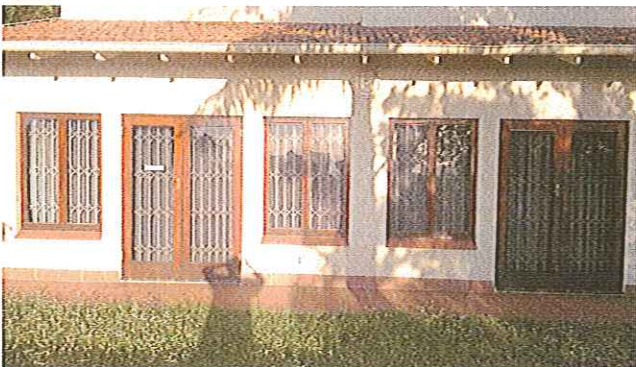
East Elevation – LHS Ground Floor
