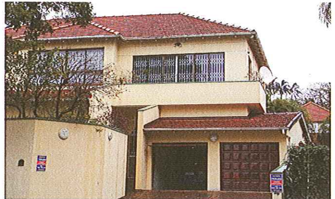
RHS of East Elevation
