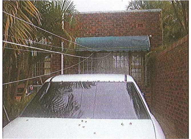
East Elevation - RHS of Outbuilding
