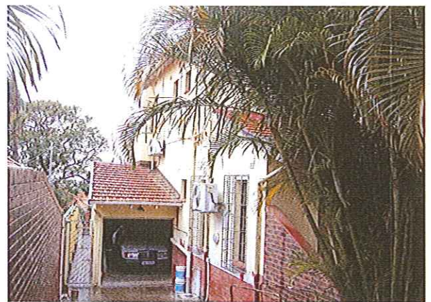
RHS of West Elevation
