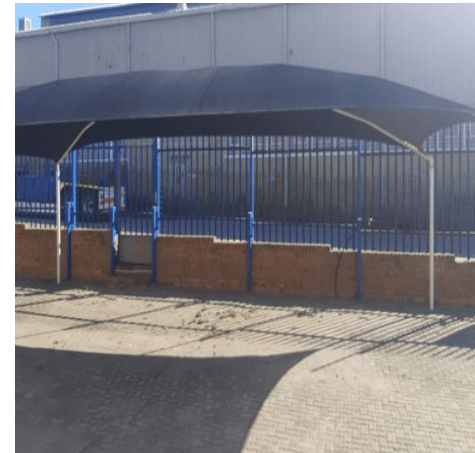
Parking area The whole site is already paved.
