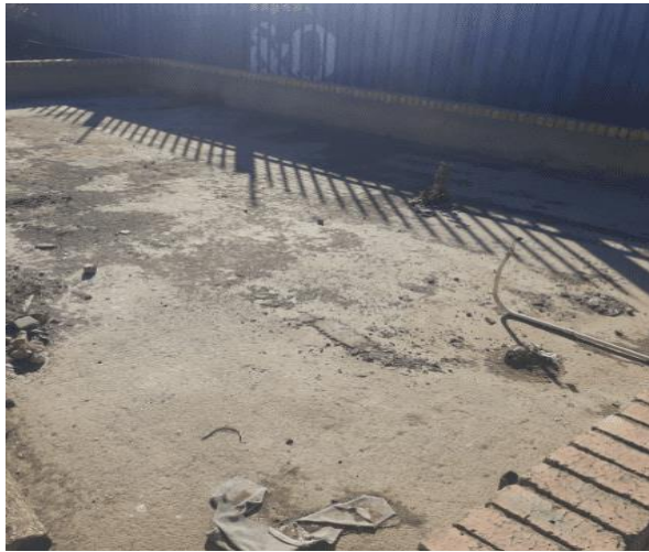
Bunding area for fuel storage already in place
