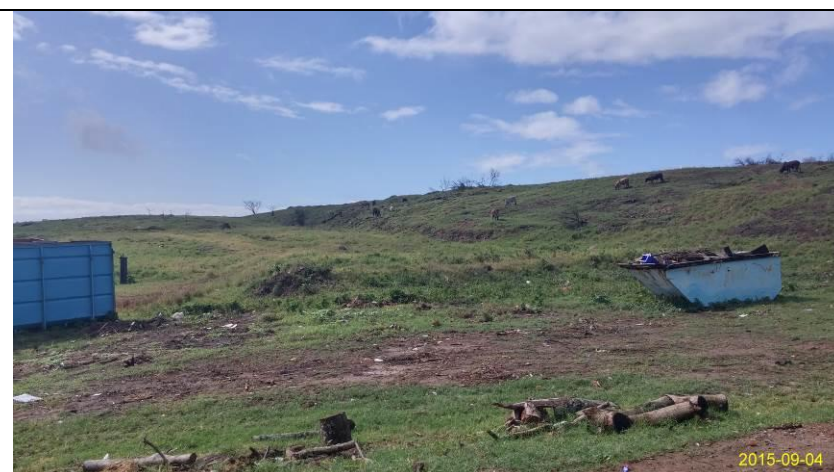
Looking east. Photograph taken near Position 2. Decommissioned landfill. Note the stormwater diversion channel. Cows have entered the site for grazing.
