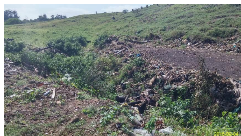
Looking east. Photograph taken near Position 2. Decommissioned landfill. Note the stormwater diversion channel at the foot of the landfill. This needs to be cleaned and maintained.
