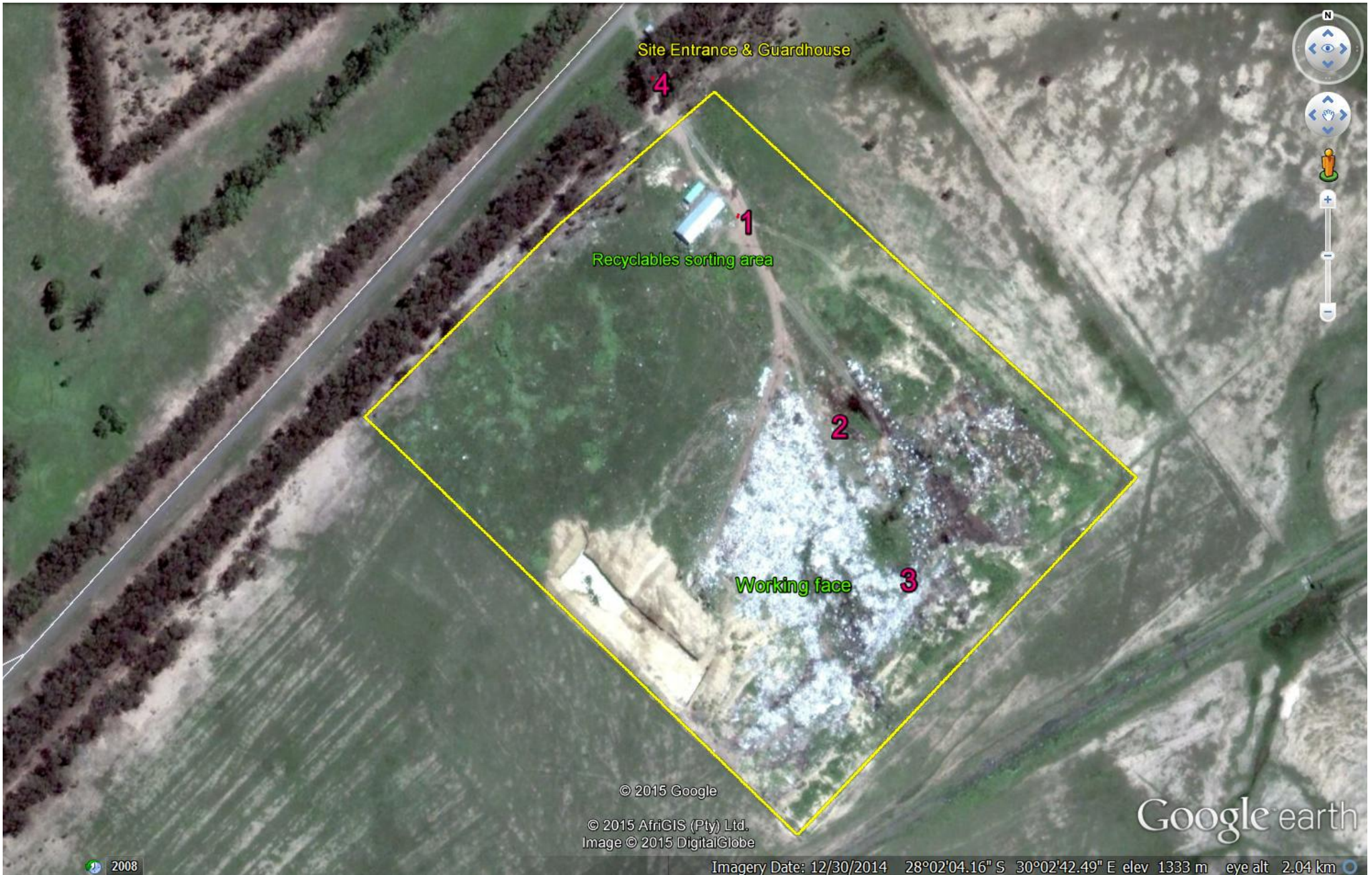
Google Earth satellite image of the Dannhauser Waste Facility and its site elements and photo viewpoints
