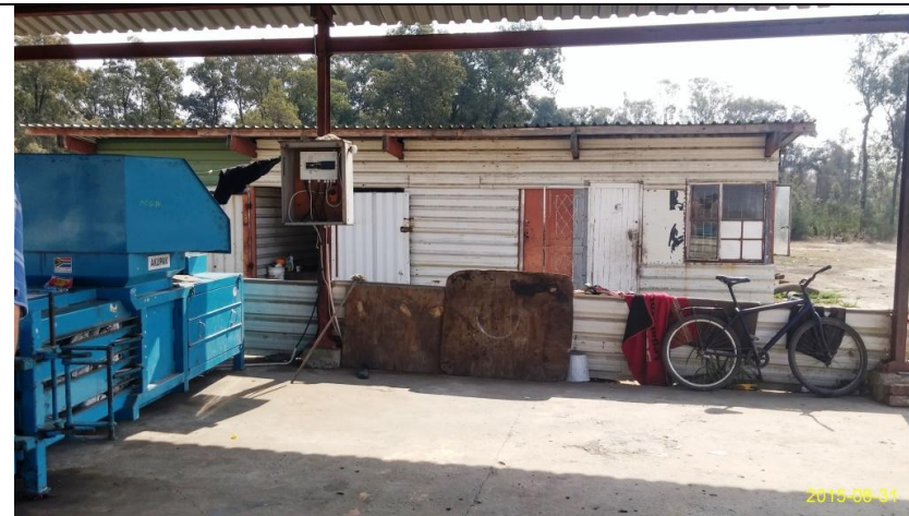
Looking north. Recyclables sorting area, baler machine on left. Photograph taken near Position 1.
