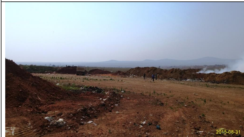
Looking north-east. Trench soil stockpiles. Photograph taken near Position 1.
