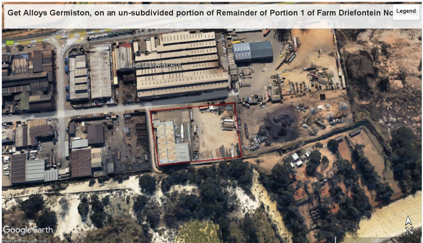
Figure 1: The un-subdivided portion of Remainder of Portion 1 of farm Driefontein No. 87-IR: Site Locality
