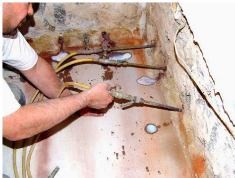
Chemical injected under pressure
