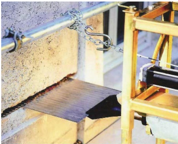
Metal plates insertion by compressed air driven jackhammer
