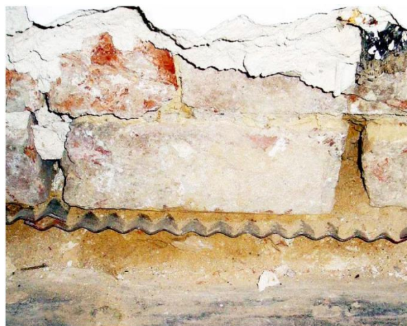
Metal plates installed at the base of a building
