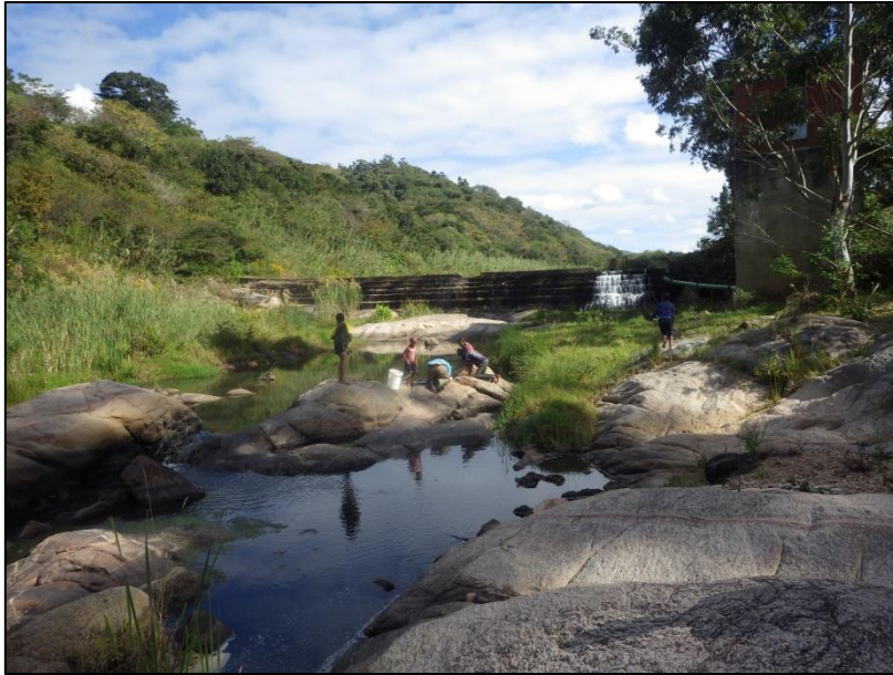
Figure 5-1: Flow Regulation, abstraction, Channel and bed Modification (A1; May 2018)
