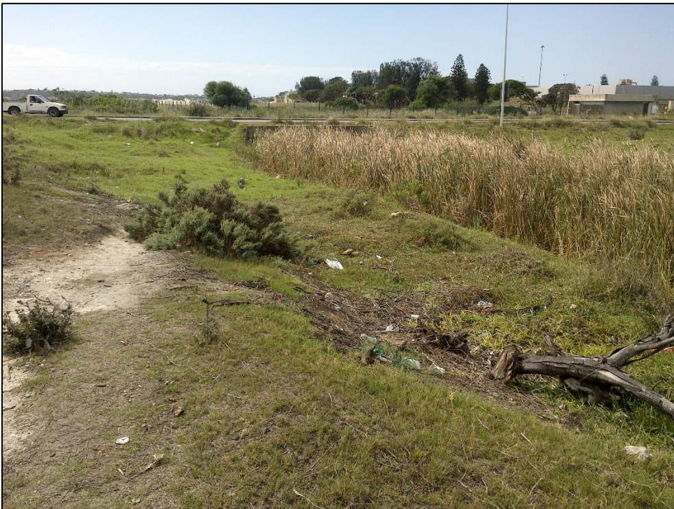
Figure 16. View of the bridge at the south-eastern corner of Grahamstown Road and John Tallant Road that will be upgraded.
