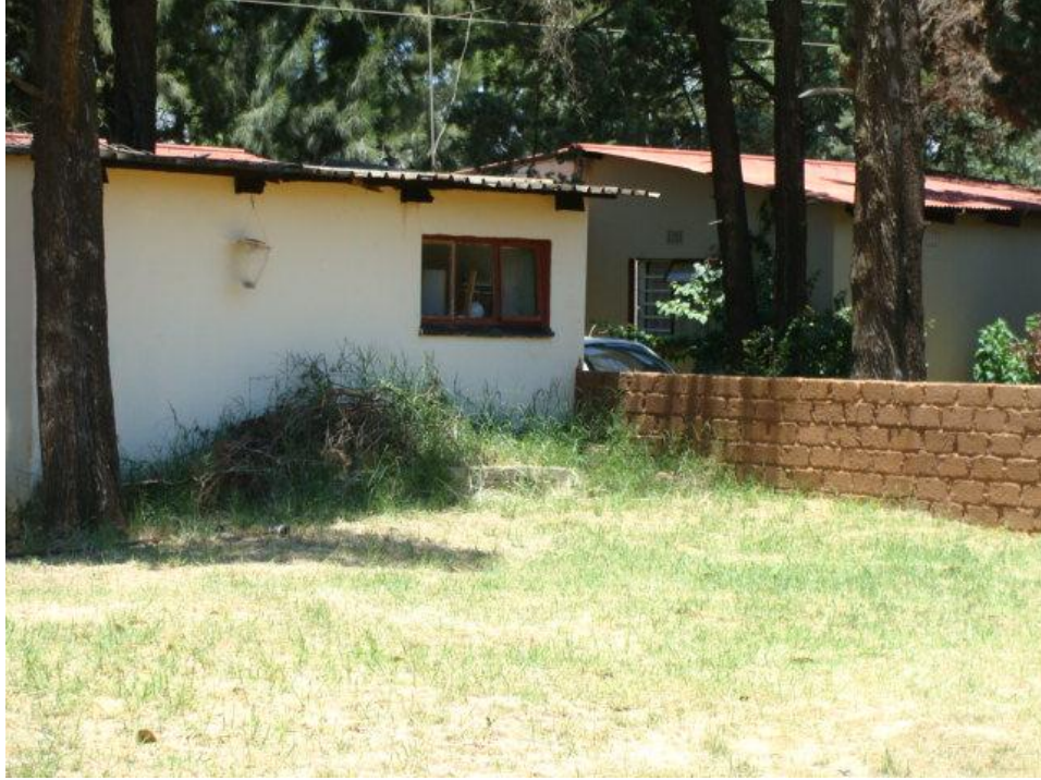
Figure 2 View of some of the buildings on site.
