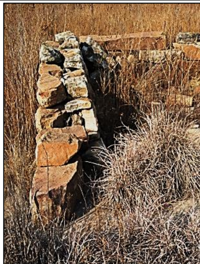
Figure 13. Section of the sandstone walling of the stock kraal (Photograph: M. Naude 2013)
