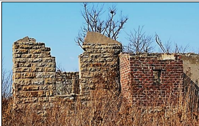
Figure 6. Small remnant of the front gable (Photograph: M. Naude 2013).
