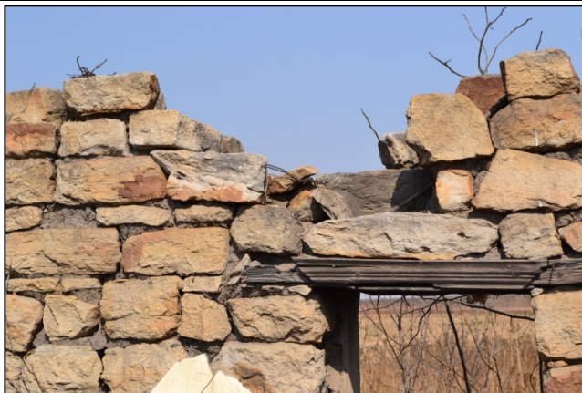
Figure 11. Detail of window lintel with architrave strip on top, still intact (Photograph: M. Naude 2013)
