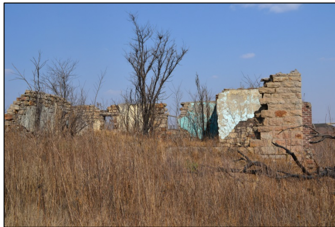
Figure 2. Remains of the front facade of the dwelling (Photograph: M. Naude 2013)
