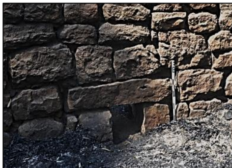
Figure 6. Water drain along the lower wall of the kraal with narrow stone lintel.
