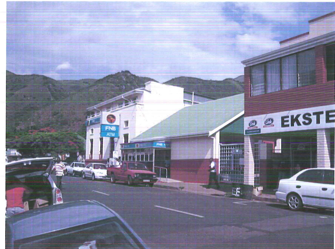
CROWN EAST FAÇADE
