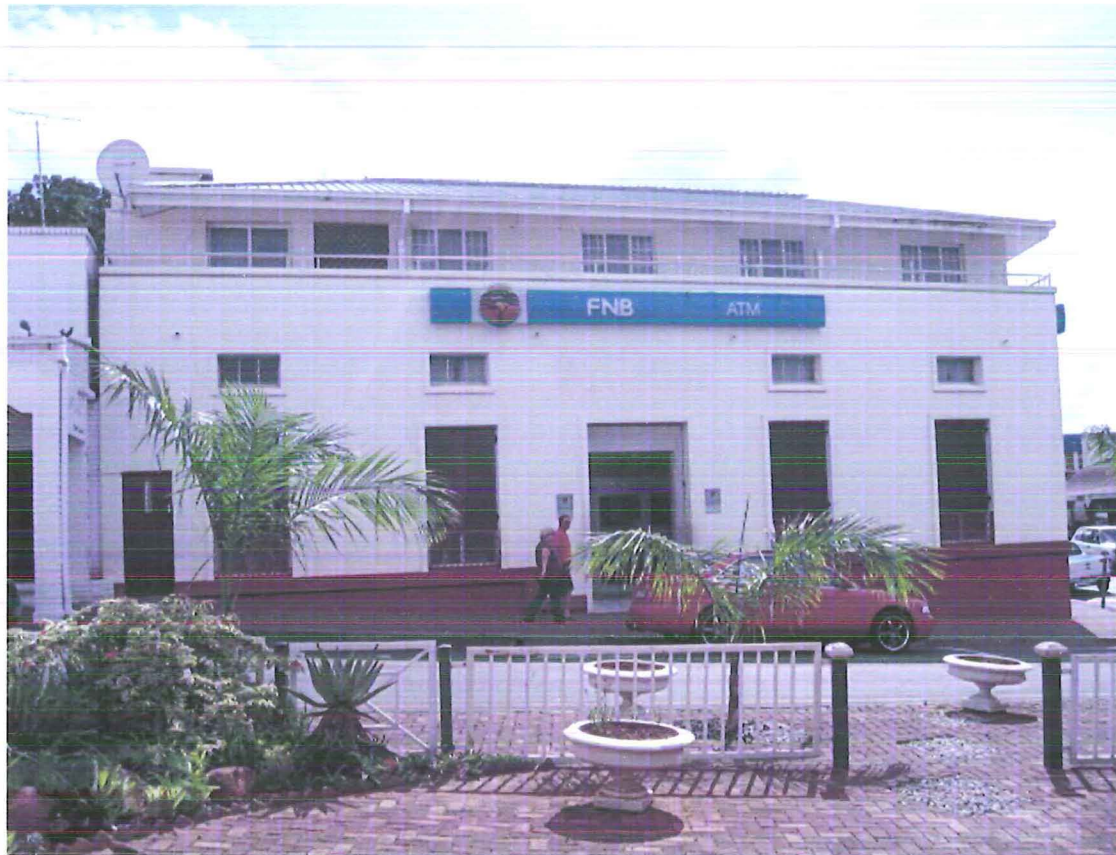
MARKET STREET FAÇADE
